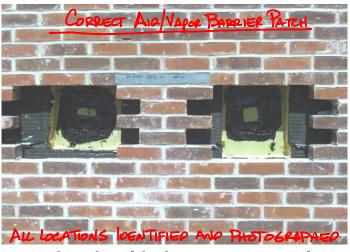
Make sure that these "tiebacks" are discussed early with the mason, exterior sheathing, and air/vapor barrier Contractor's...with the understanding of proper correction to the substrates, including overlaps, room for re-installation, etc.
